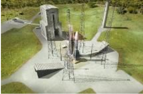
Newly developed Launch Zone Mobile Gantry: 100 meters high, 5.000 t
