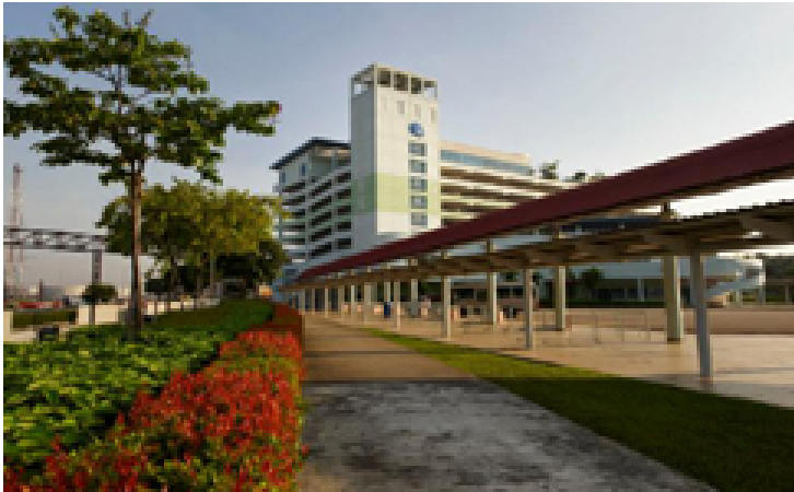
Amenity Facility - Sakra Oasis with Carparks
