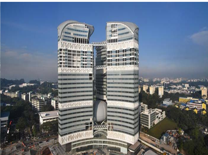
Fusionopolis One – largest steel building project for JTC during its conception. Its unique design consists of 3 high-rise towers (Symbiosis 22 storeys, Connexis North 24 storeys and Connexis South 21 storeys) linked by sky bridges alongside an Experimental Theatre supported at six stories above ground perched above a single column support.
