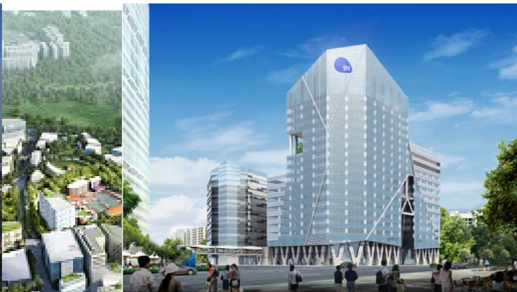
Fusionopolis Two – comprising 3 towers of total 103,635 sqm space, features Singapore's largest multi-storey R&D clean room facility and is designed with stringent micro-vibration requirement of VC-E at Tower C.
