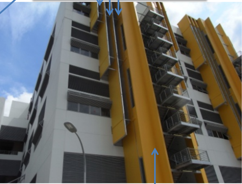
Stacks with pre-installed gravity flow down pipes with low resistance for customers to discharge segregated industrial wastewater directly to the CWTP
