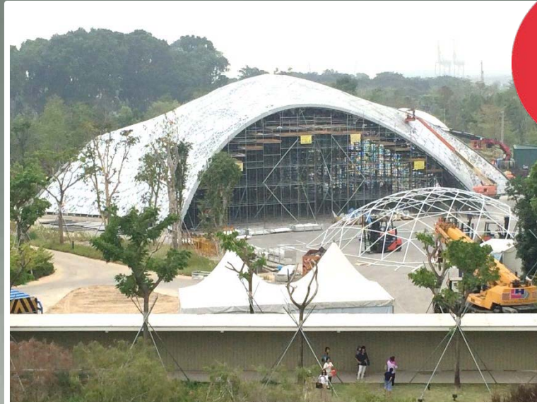
SG 50 EXPO PAVILION @ MARINA BAY (opening 15-11-15)
